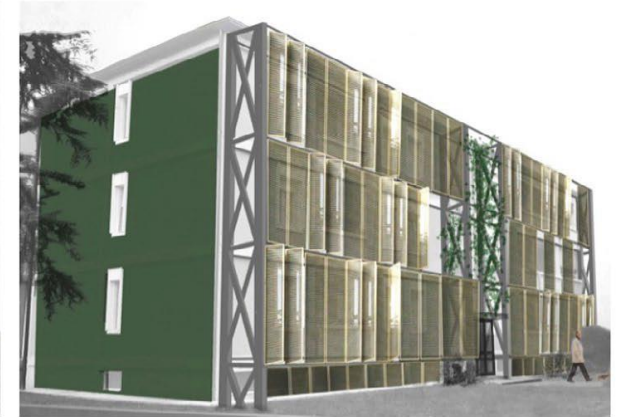
Integrated steel-braced shear wall exoskeleton Bellini et al. (2018)
