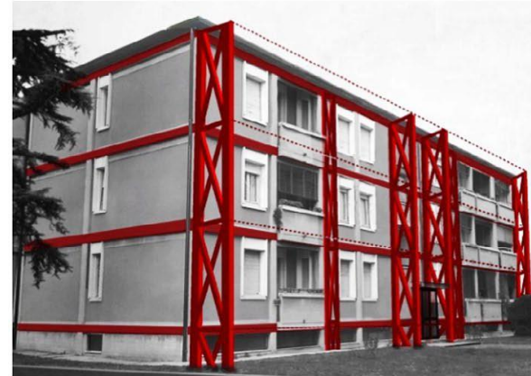
Integrated steel-braced shear wall exoskeleton Bellini et al. (2018)
